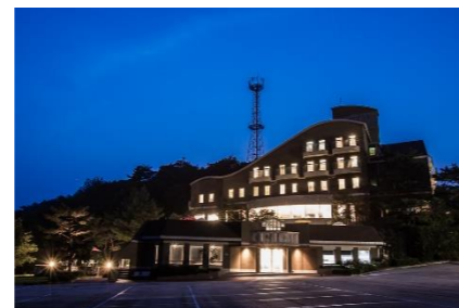
Nepes Training Center View of Hotel West of Canaan
